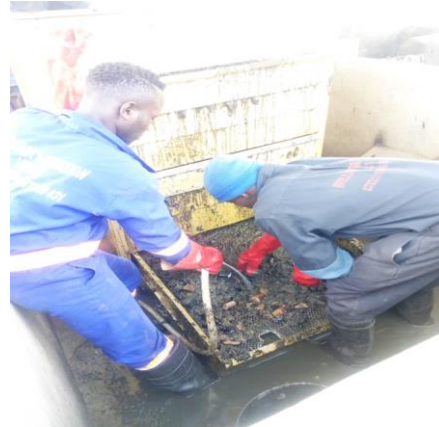
Figure 3-7: solid waste retained on sieve being washed further
