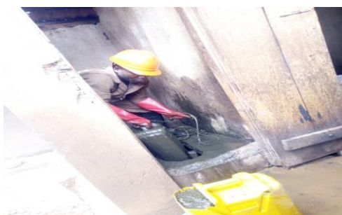
Figure 3-3: a worker manually empties the contents of the pit
